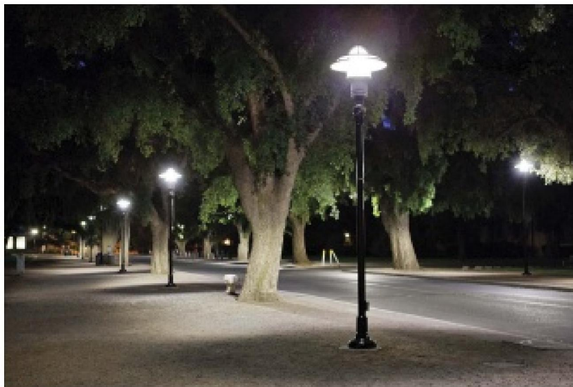
FIG. 2. Networked LED-based post-top lighting at the University of California at Davis.
